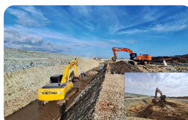
Construction of Spillway Downstream Channel
