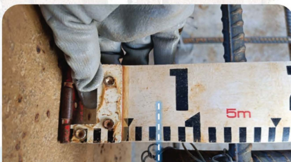
Checking the concrete cover concrete cover Actual = 75 mm
