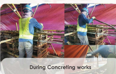
Checking of Anchor Bolt Alignment
